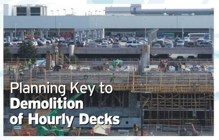
Work on the back half of the new Hourly deck is currently underway. In January, crews will begin building the front half, but first CLT must tear down the current Hourly decks and relocate Queen Charlotte to make room.
