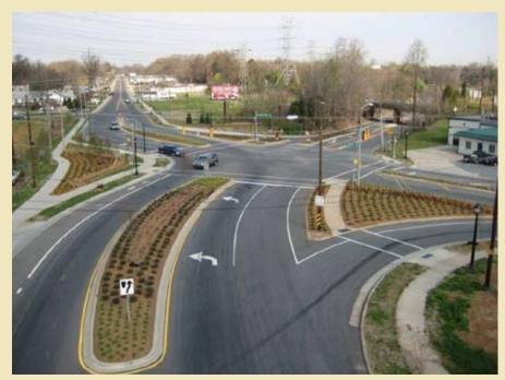
The picture above illustrates an example of using Complete Streets design concepts to accommodate several modes of transportation in a unique, and challenging, situation. At this intersection, pedestrian crossings have been shortened, bicycle and pedestrian spaces are more visible, and traffic flow has not been impeded.
