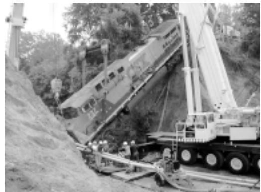
Figure 2: Flooding has caused significant property damage throughout Mecklenburg County. In this photo, a CSX railroad engine is pulled from Little Sugar Creek after floodwaters washed out the railroad bridge supports.
