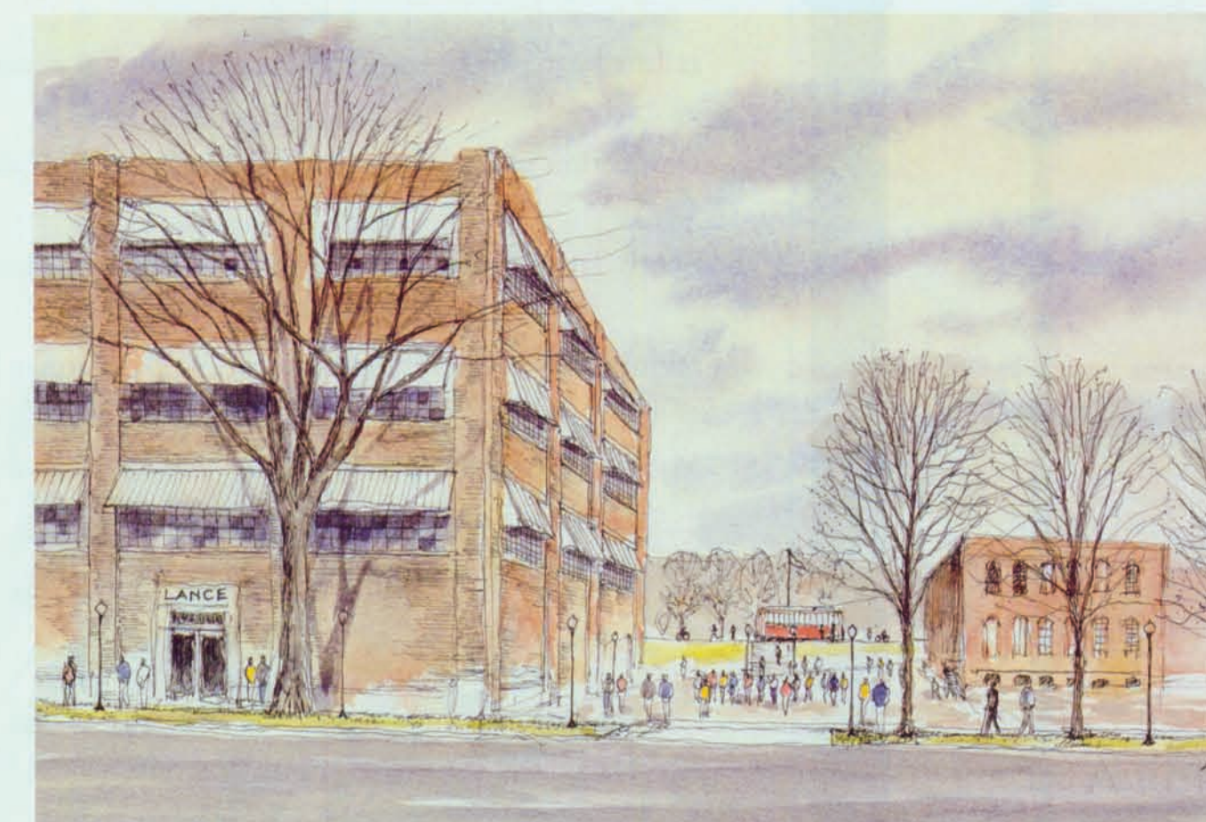
Lance and Park Elevator Buildings
