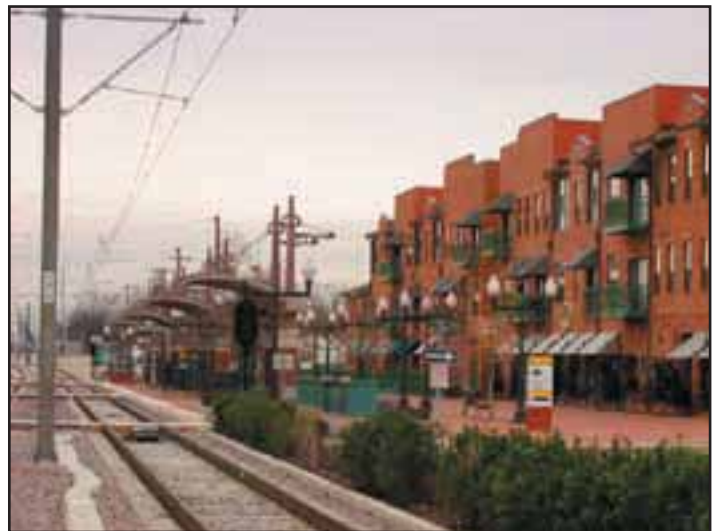
Mixed-use development fronting Dallas light rail line
