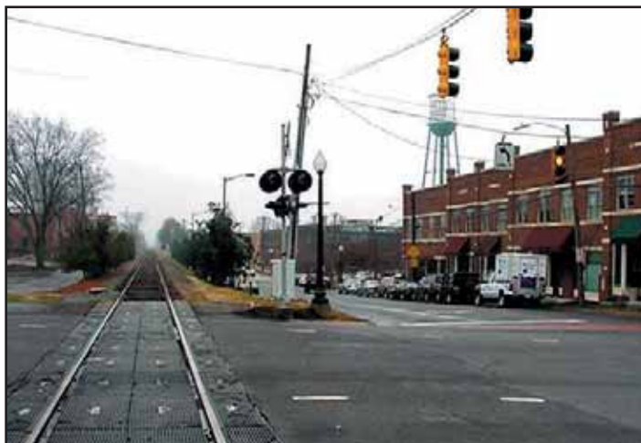
Camden Road and Rail Line at East Boulevard
