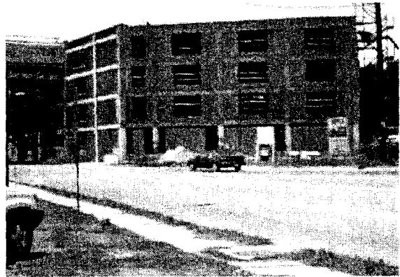
1230 West Morehead – new offices in a redeveloped structure.
