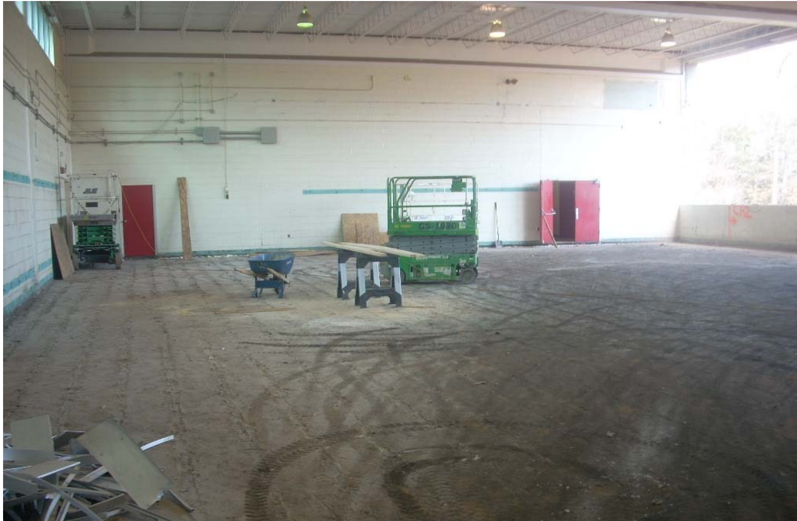
Alexander Graham Middle School Gym Renovation/Addition
