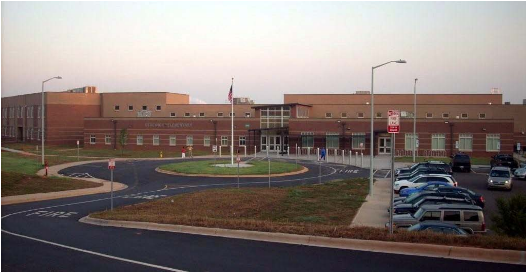
Berewick Elementary School (E07-01) Front Entrance
