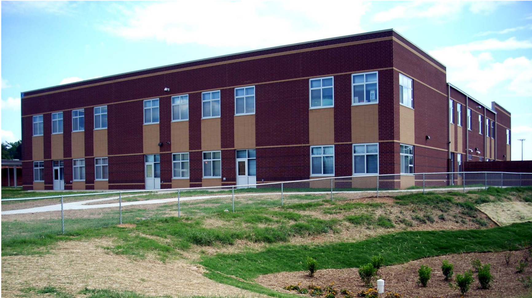
North Mecklenburg High School New Classroom Building
