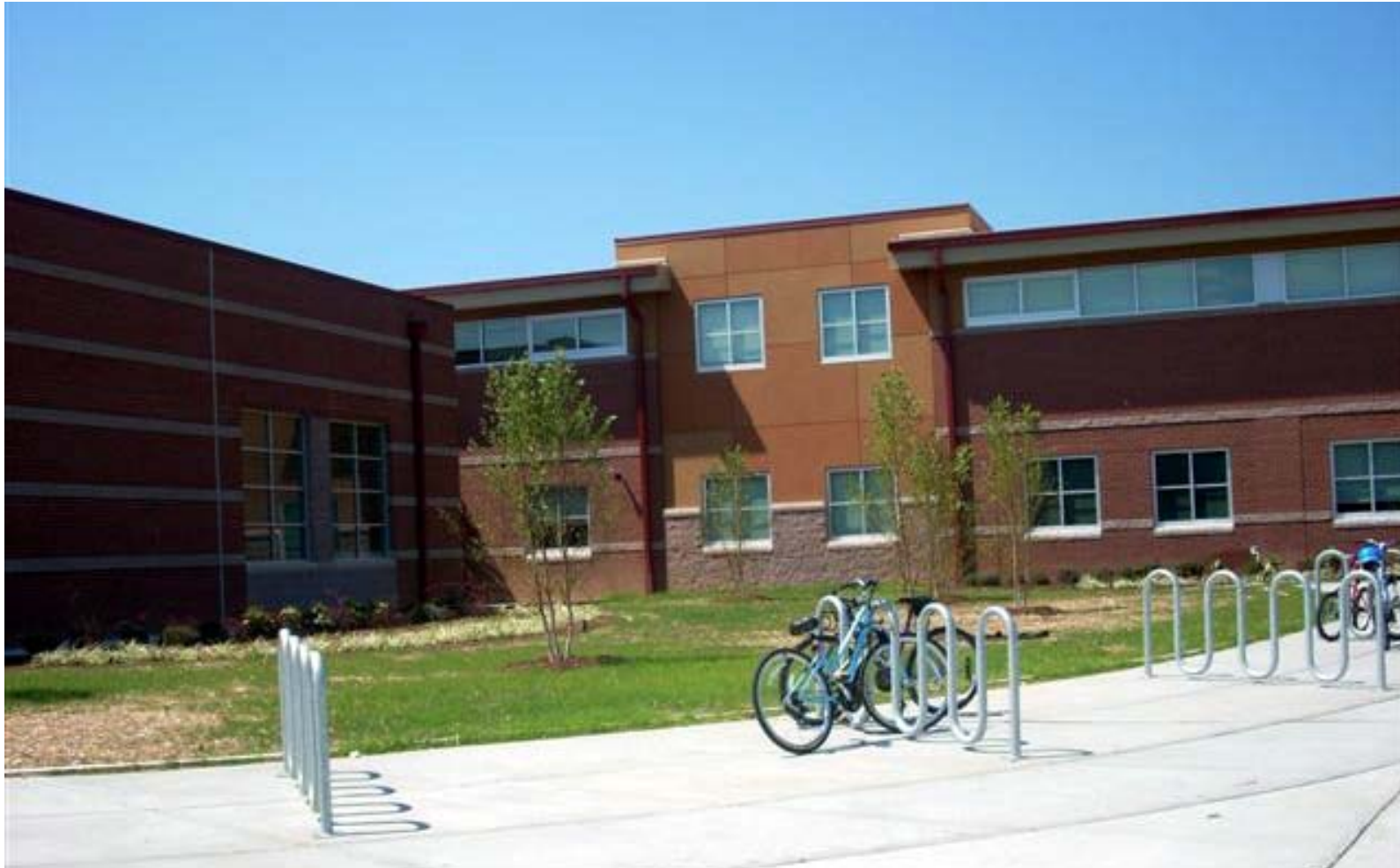
Ridge Road Middle School Main Entrance
