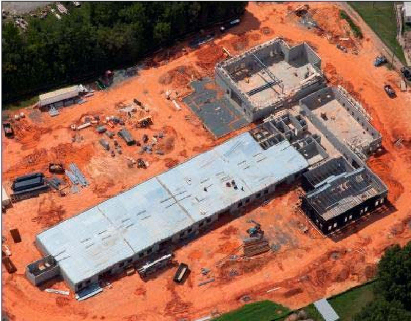
Bain Elementary School Replacement School
