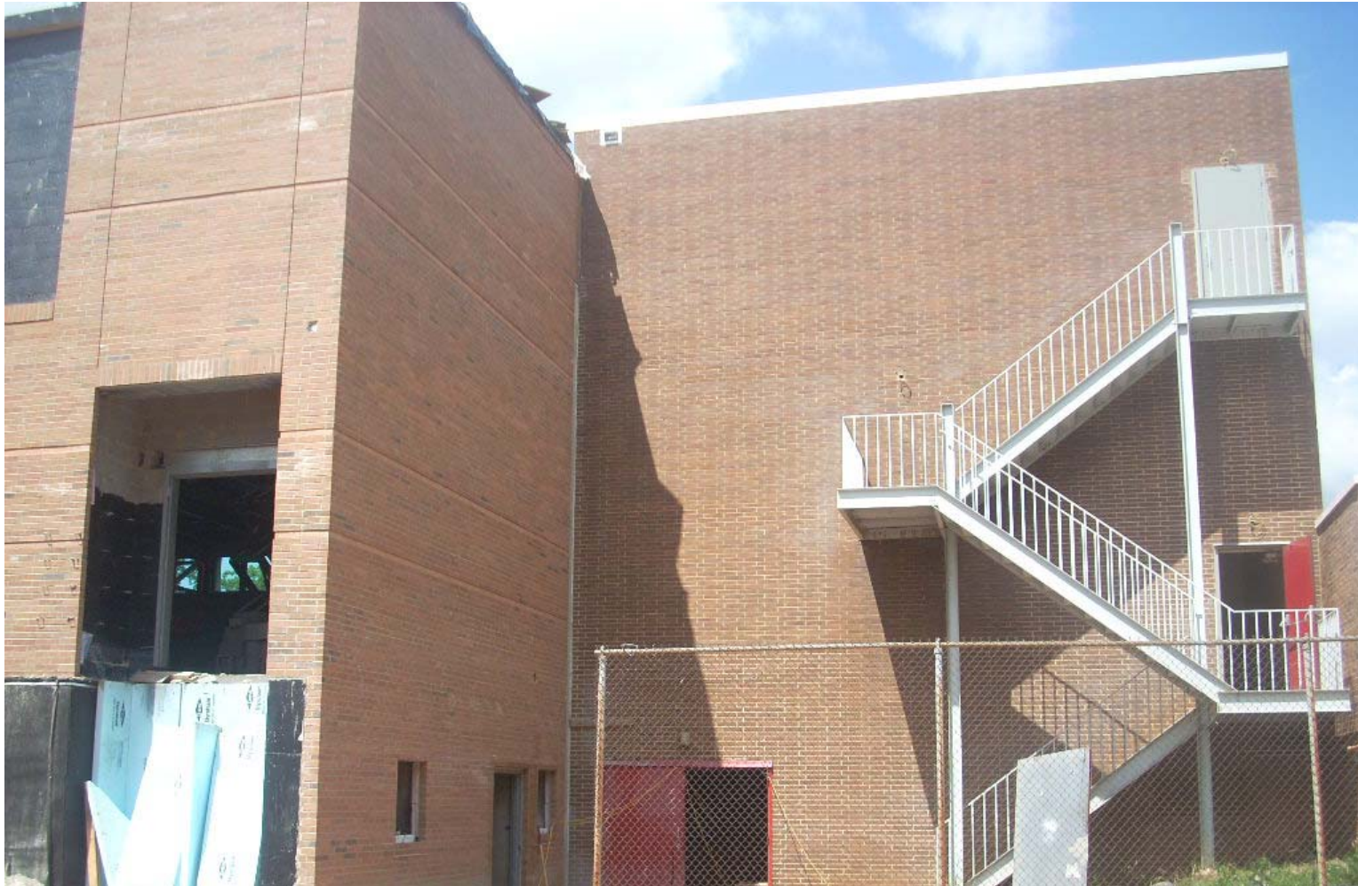
Alexander Graham Middle School Gym Renovation/Addition
