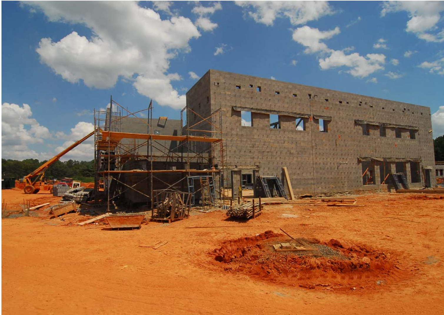
Bain Elementary School Replacement School
