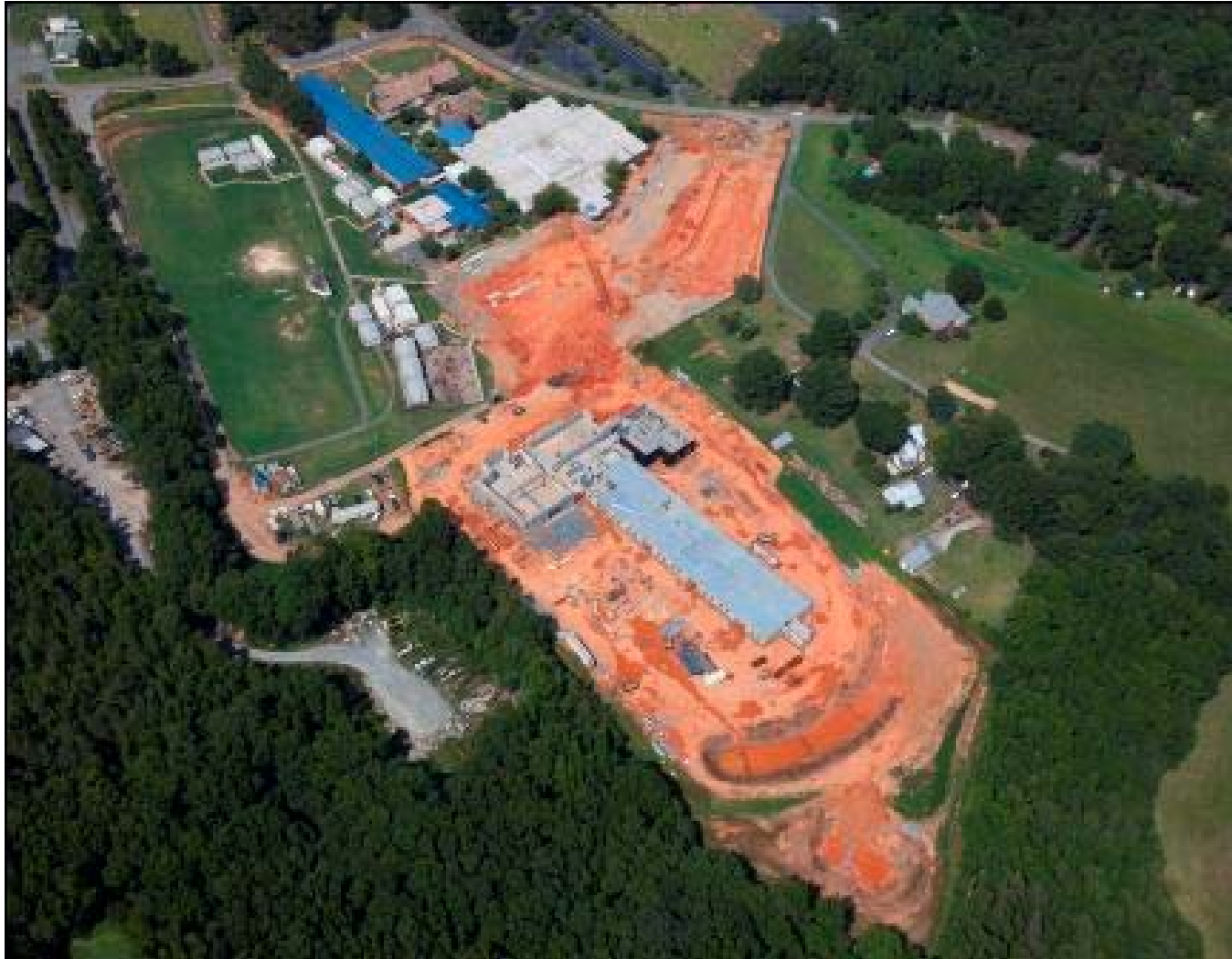
Bain Elementary School Replacement School
