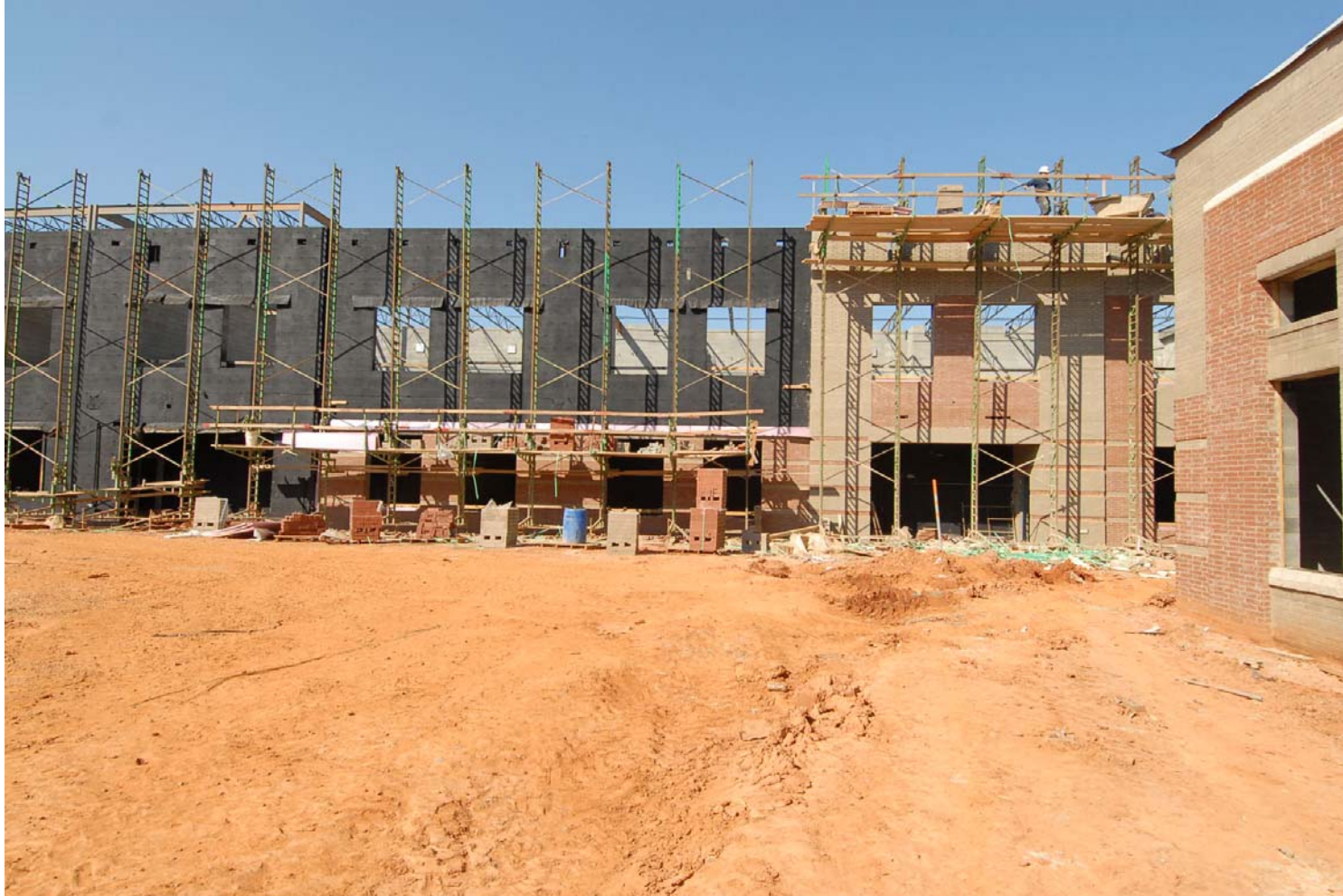
Bain Elementary School Replacement School
