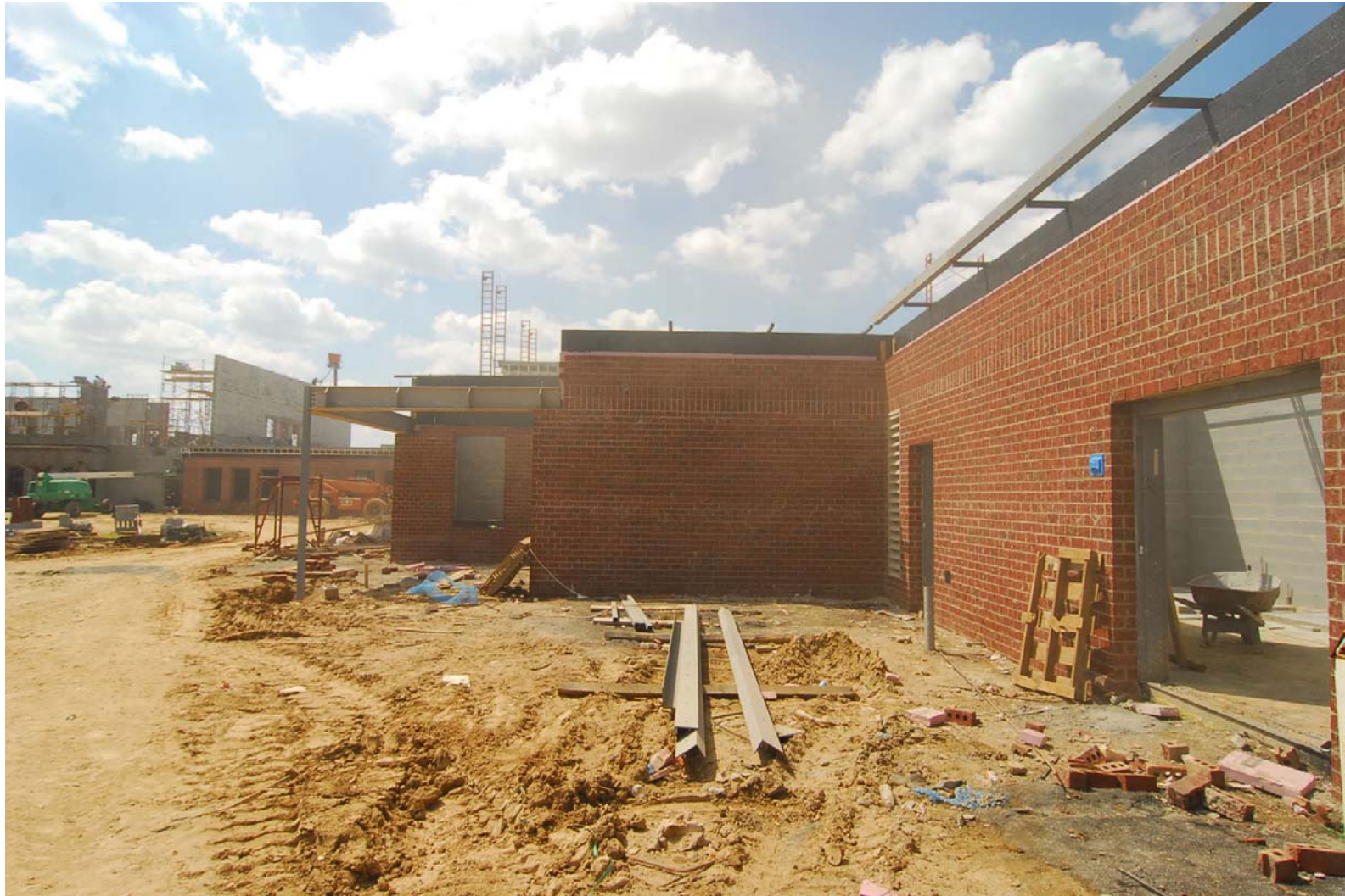
Pineville Elementary School Replacement School
