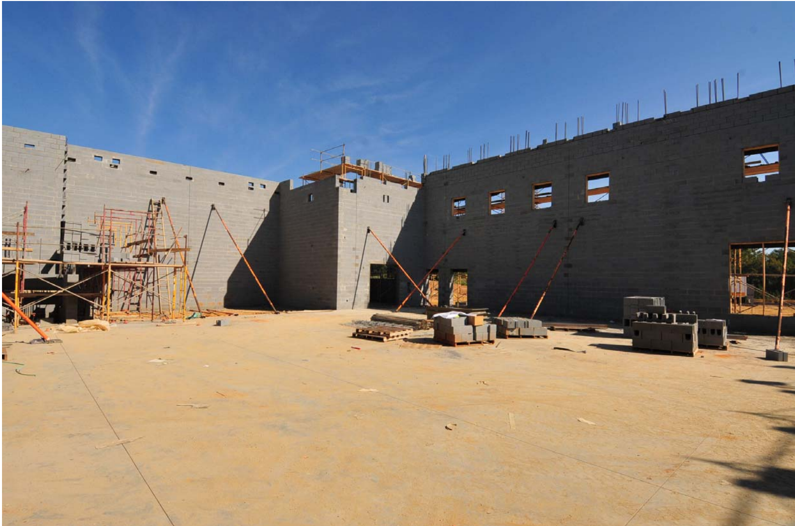
New ES (07-07) Torrence Creek Relief New Elementary School
