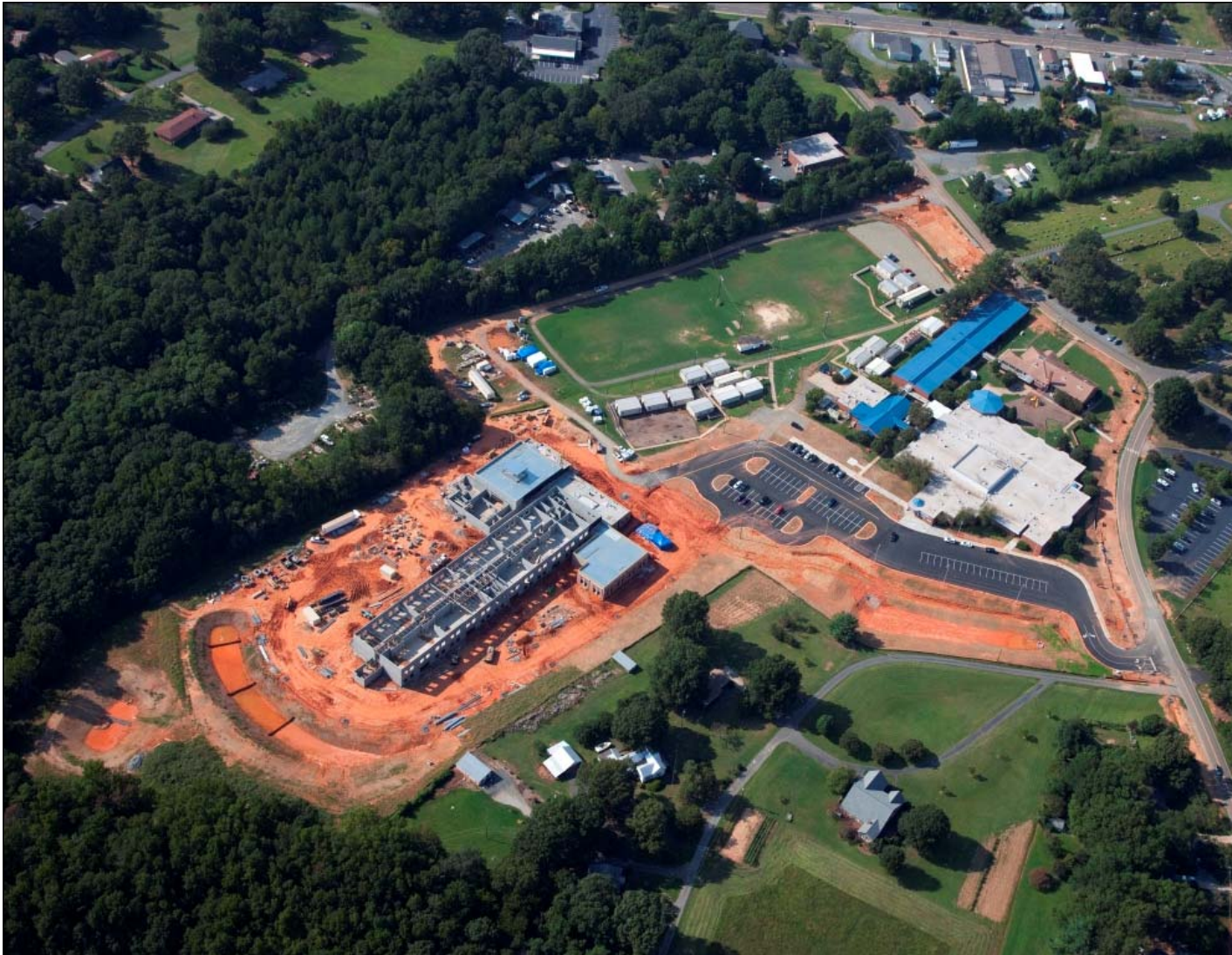
Bain Elementary School Replacement School
