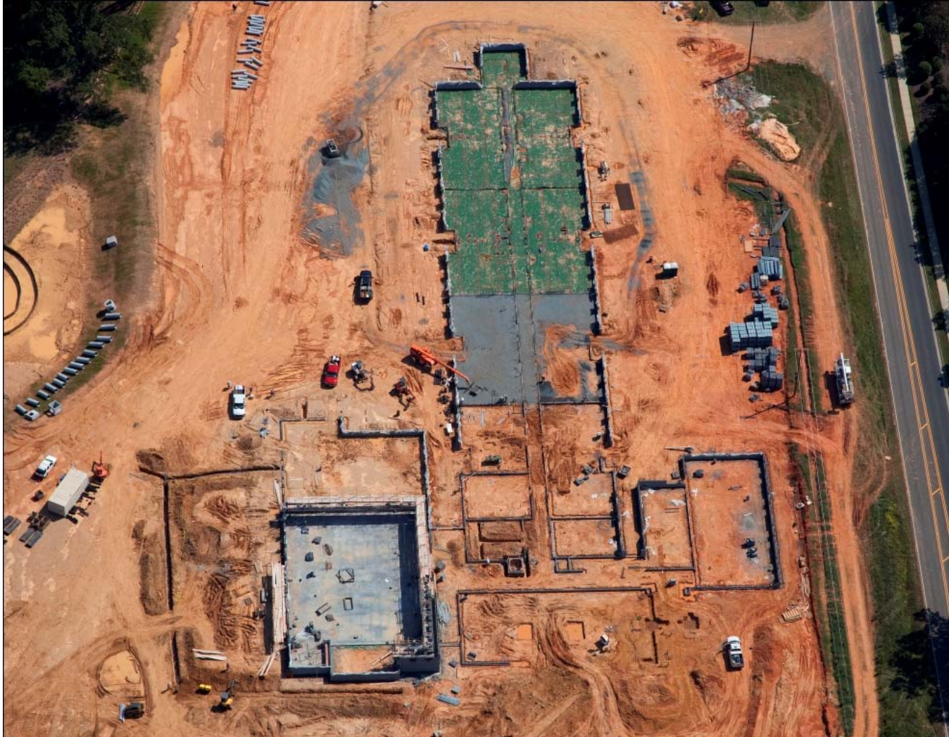
New ES (07-07) Torrence Creek Relief New Elementary School
