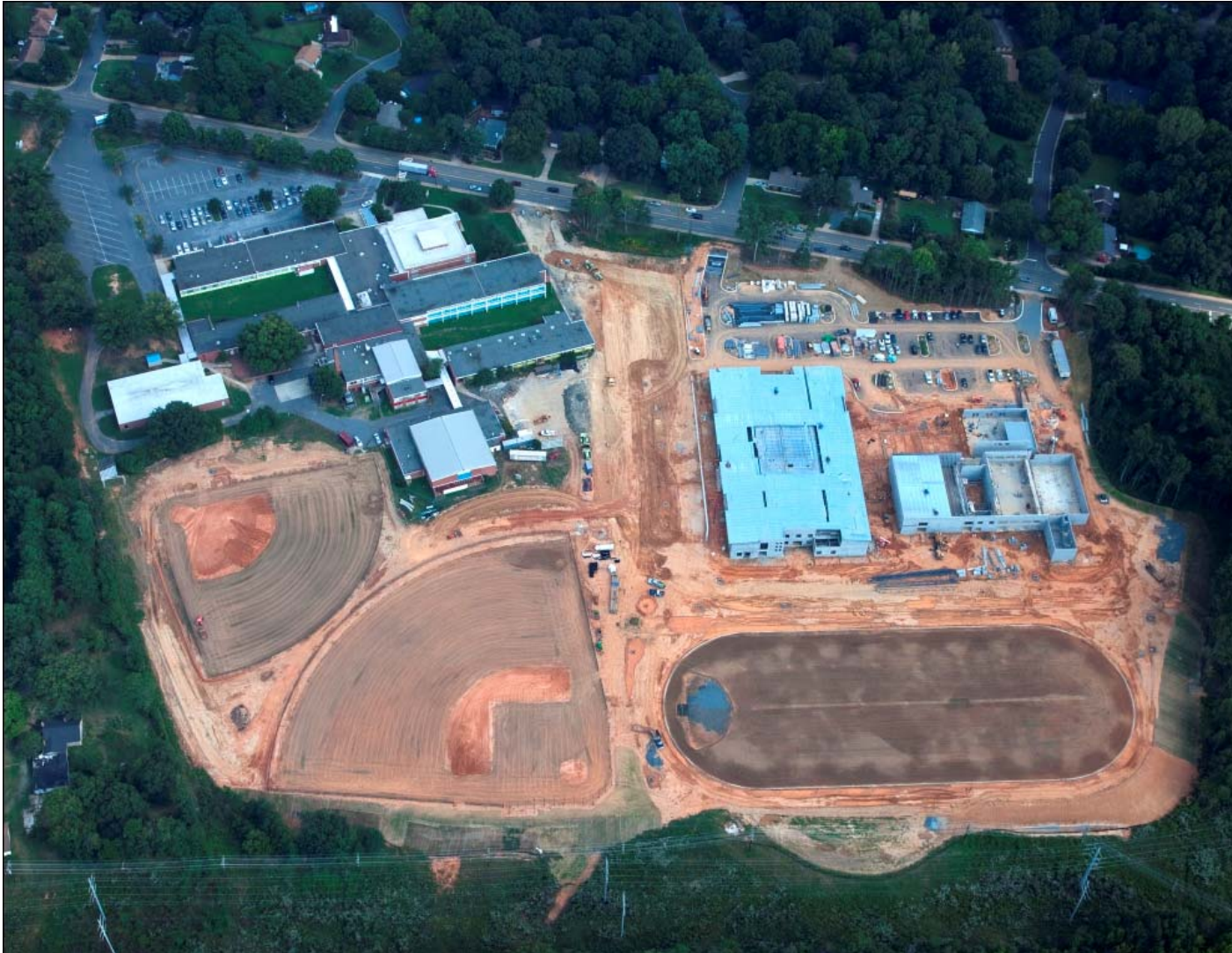
McClintock Middle School Replacement School
