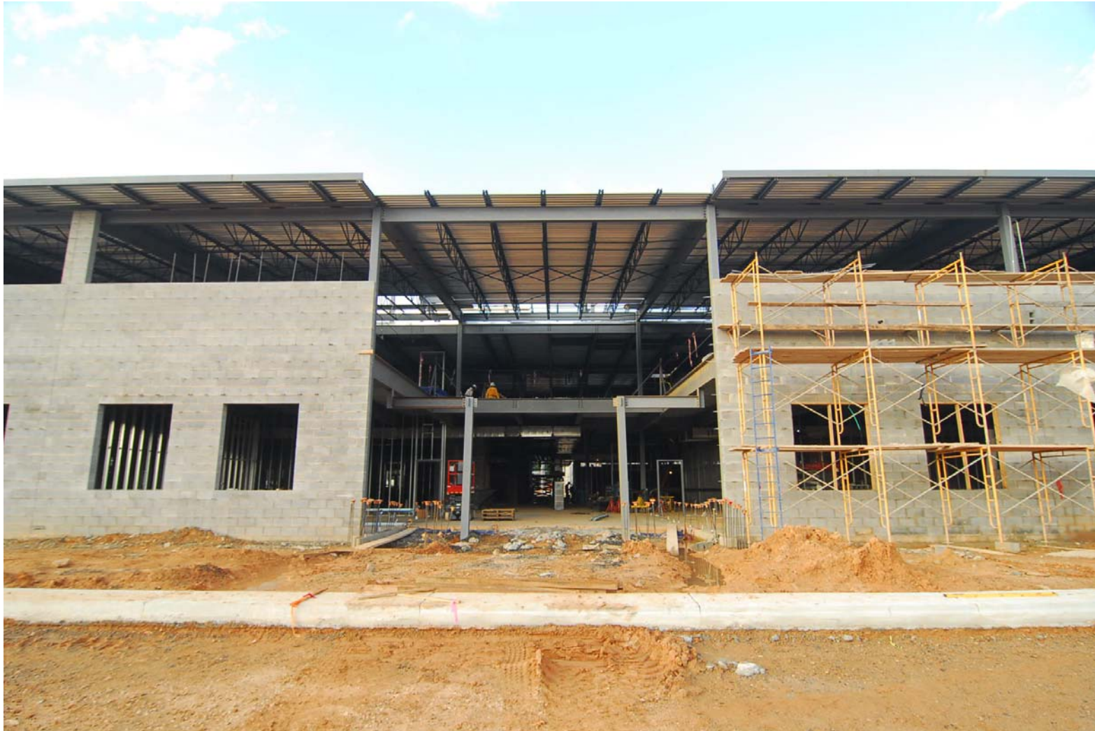
McClintock Middle School Replacement School
