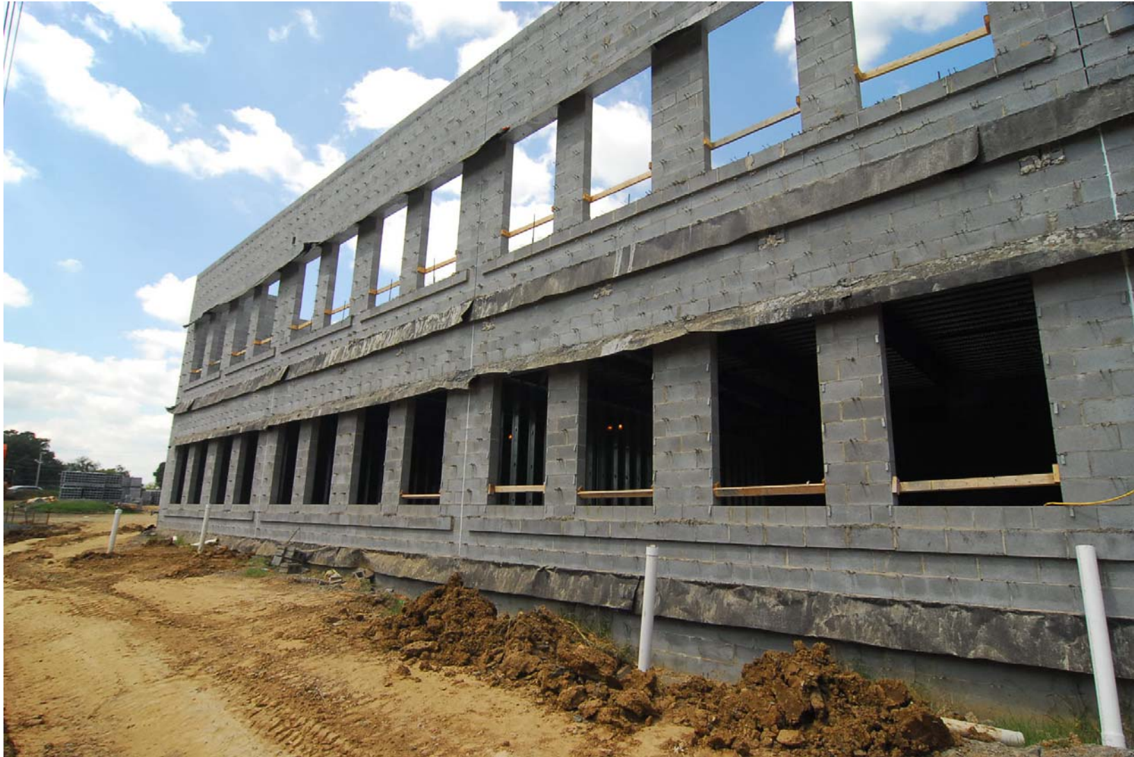
Pineville Elementary School Replacement School
