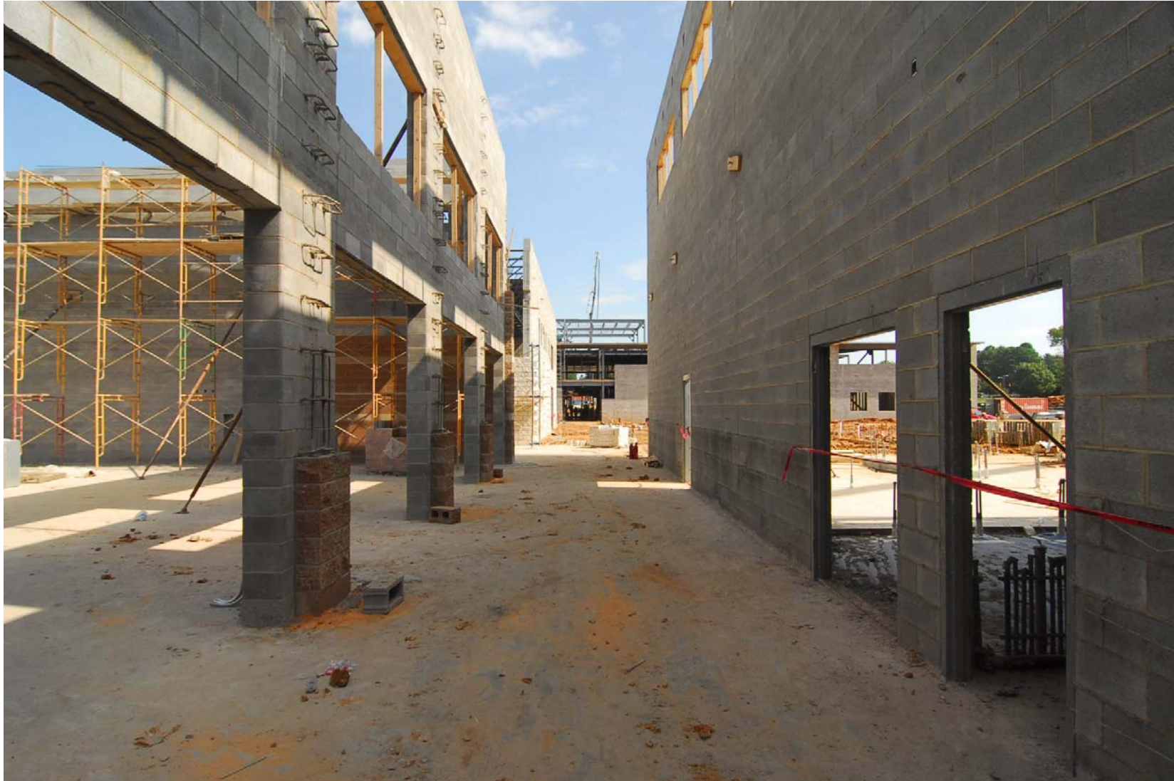
McClintock Middle School Replacement School
