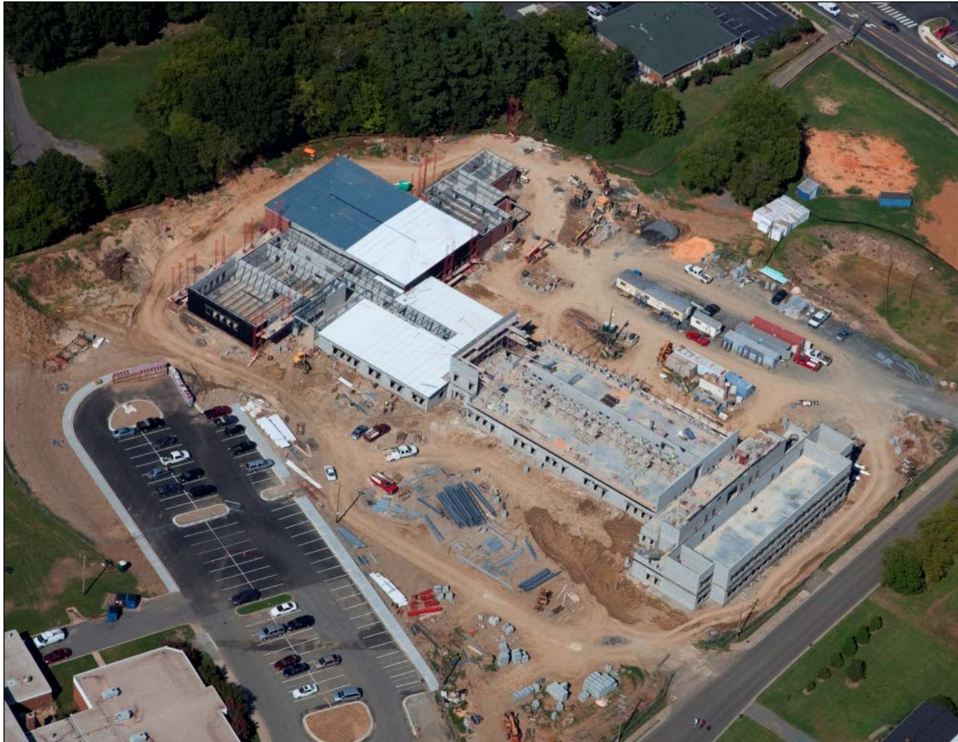
Pineville Elementary School Replacement School
