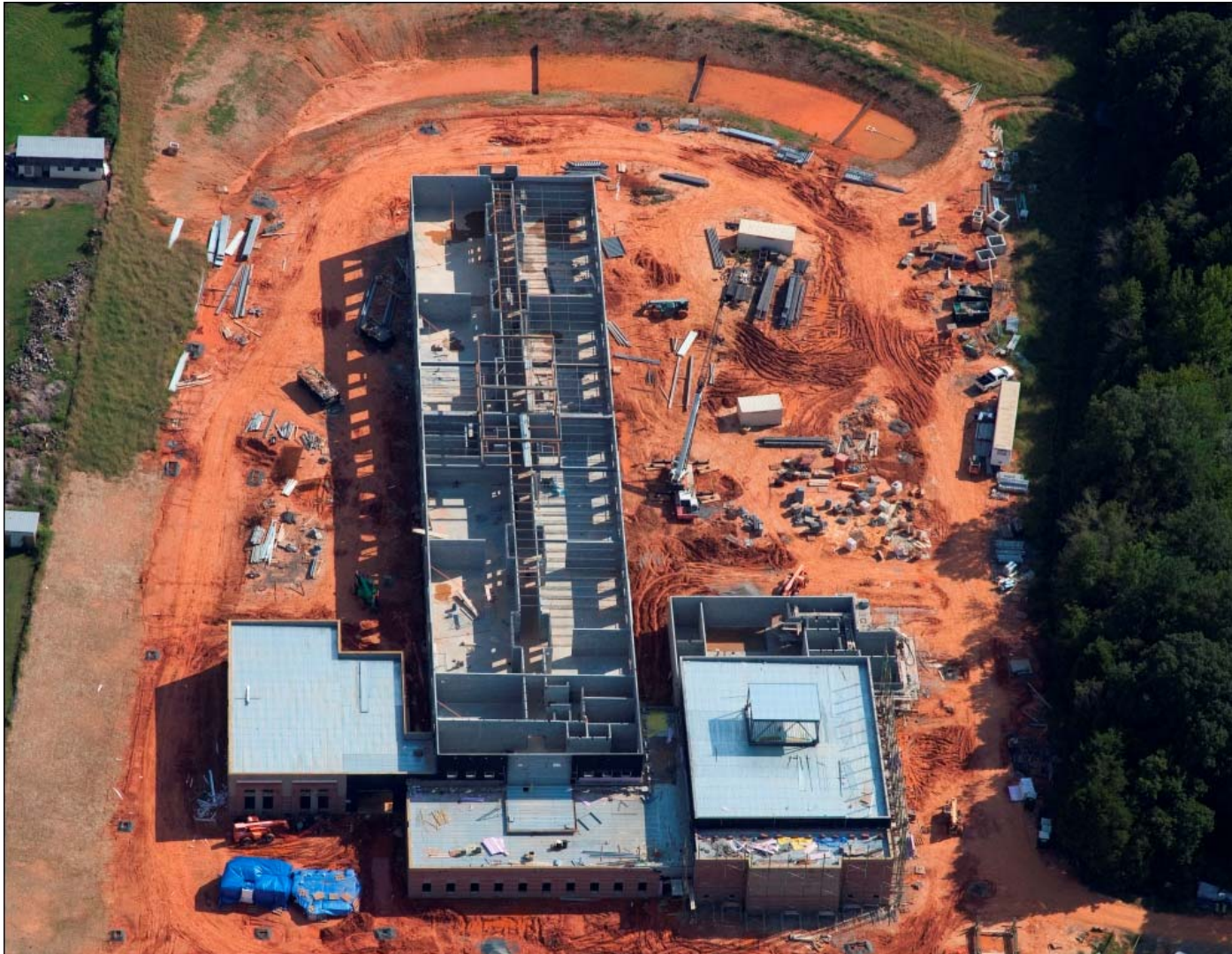
Bain Elementary School Replacement School
