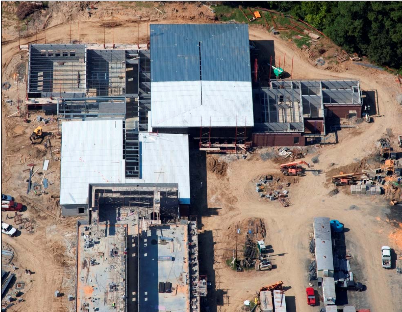
Pineville Elementary School Replacement School
