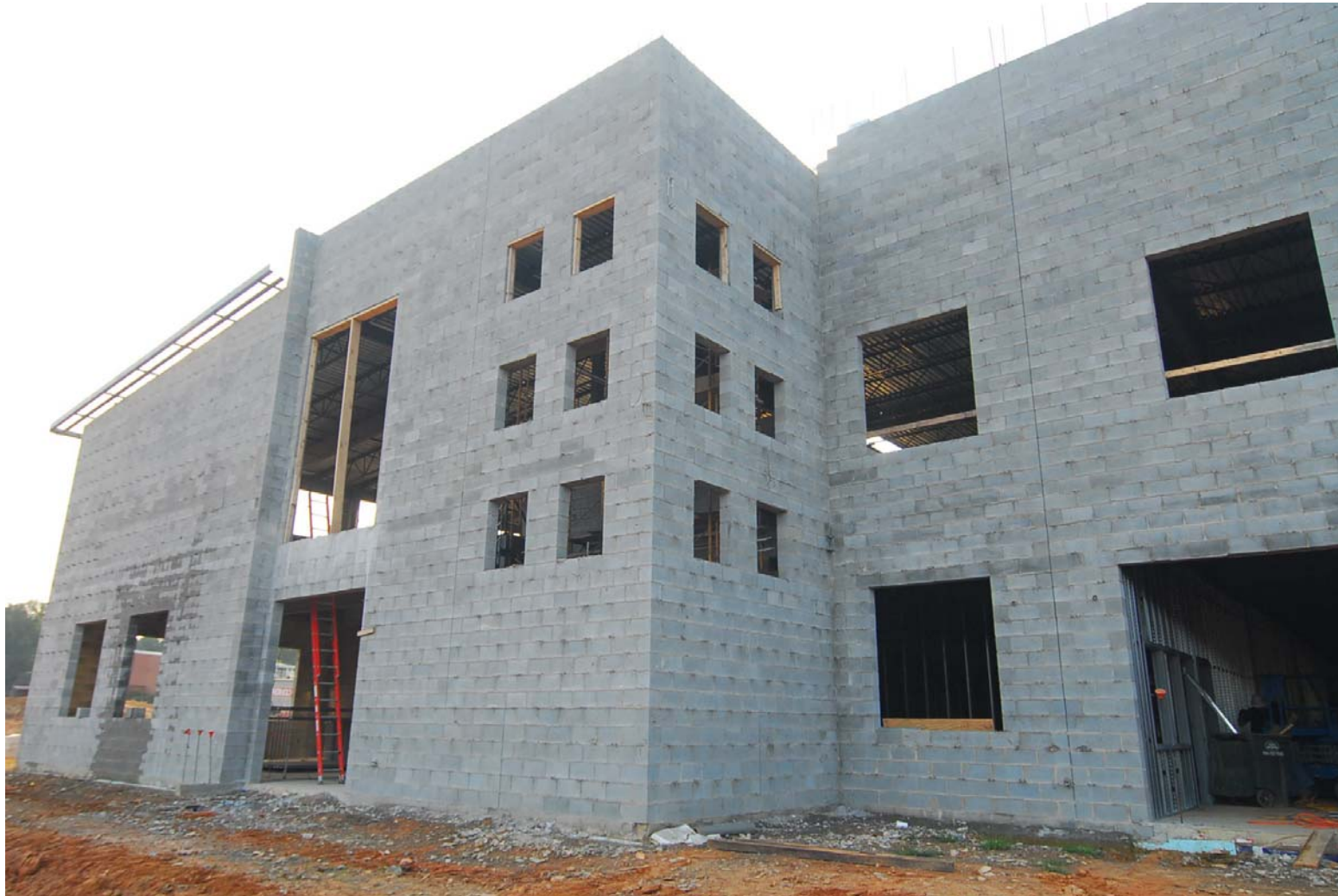
McClintock Middle School Replacement School
