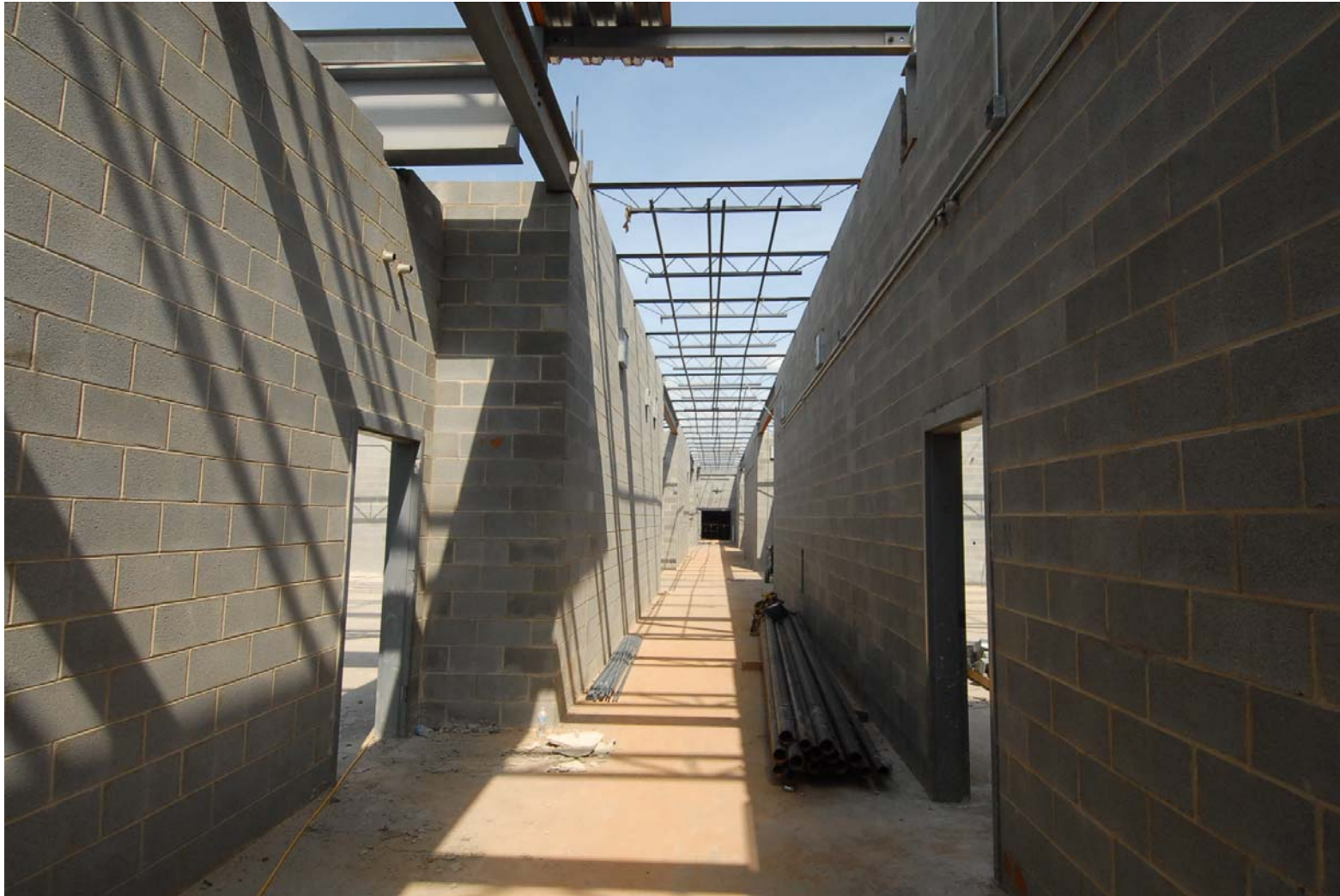
Bain Elementary School Replacement School
