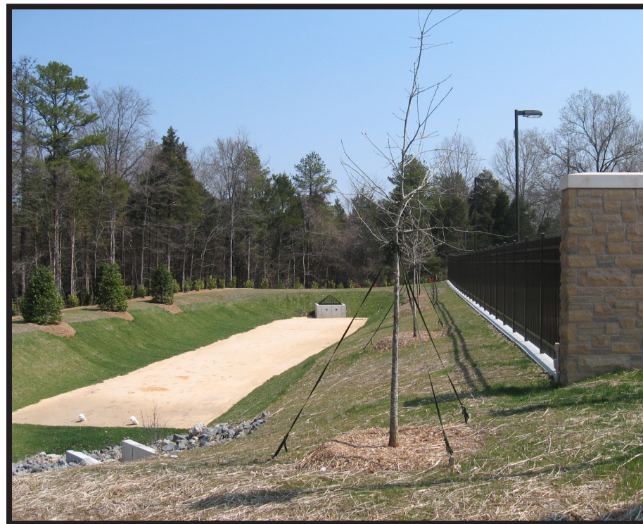
A sand filter is another type of structural BMP. This one installed at fire station #39 prevents pollutants from entering nearby streams.
