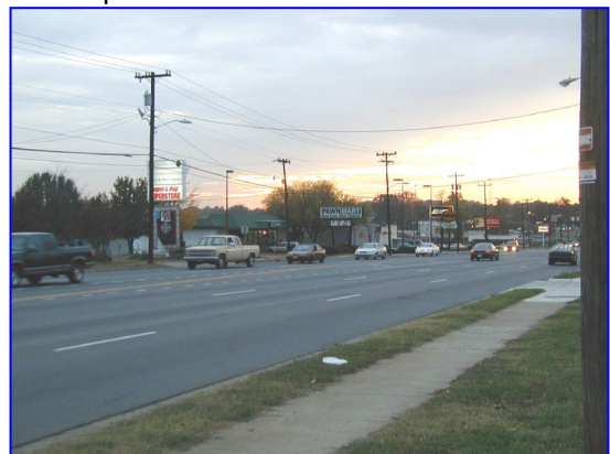
LRT in NE-5 would be within its own dedicated right of way in North Tryon Street.
