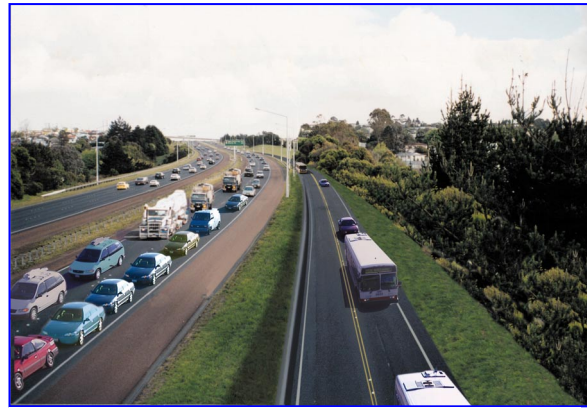
North Shore Busway – BRT in Separate Guideway
