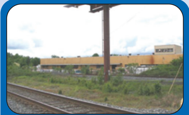
Standard Chemical Products Plant, Warehouse, East Elevation, Looking West.
