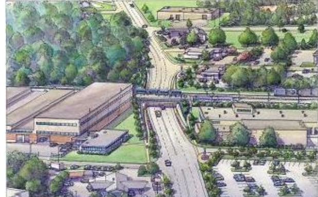
Rendering of the proposed depression of Sugar Creek Road under the existing freight tracks and proposed Light Rail Alternative.
