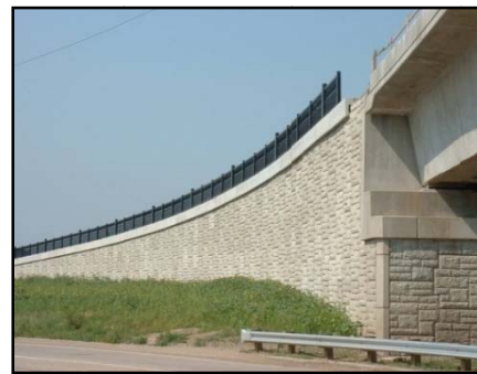
Retained fill configuration example.
