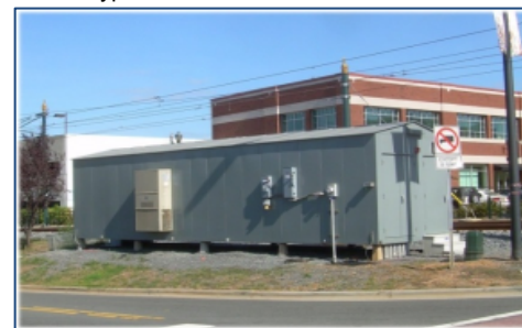
Typical LYNX Blue Line signal house.
