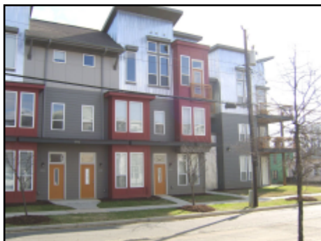
New residential construction at East 16th Street.
