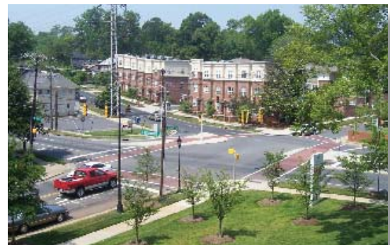
The intersection of Scott, Kenilworth, Romany and Harding was retrofitted with a left-turn lane, pedestrian-crossing islands, stamped crosswalks and countdown timers to provide a safer intersection for all travelers.
