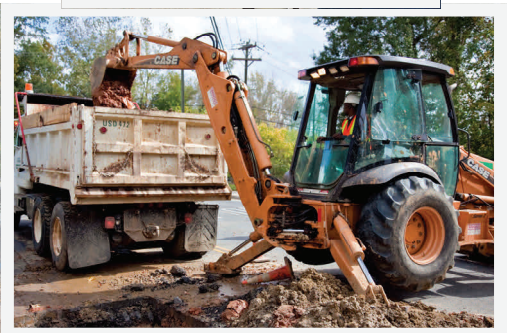
A shift from high growth focus to emphasis on system maintenance continued. CMUD faced a series of water main breaks along a stretch of 24-inch water pipe in south Charlotte, causing significant traffic problems and repair expense. After hydraulic studies deemed most of the 1970's-era pipeline no longer essential to the distribution system (thanks to infrastructure improvements of the past decade), most sections of line were retired from service over the winter.
