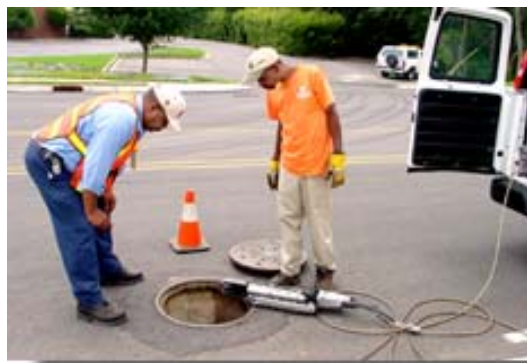
Crews use robotic cameras to check wastewater pipes
